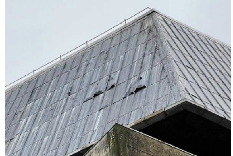
Lead faced Mansard Vertical Roof
